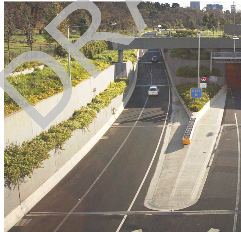
STEEP CUTTING/EMBANKMENT: BENCHING WITH PLANTING
