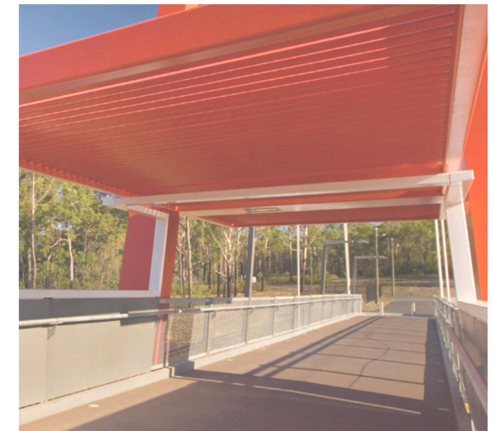
EXAMPLE OF A PEDESTRIAN BRIDGE SHADE STRUCTURE
