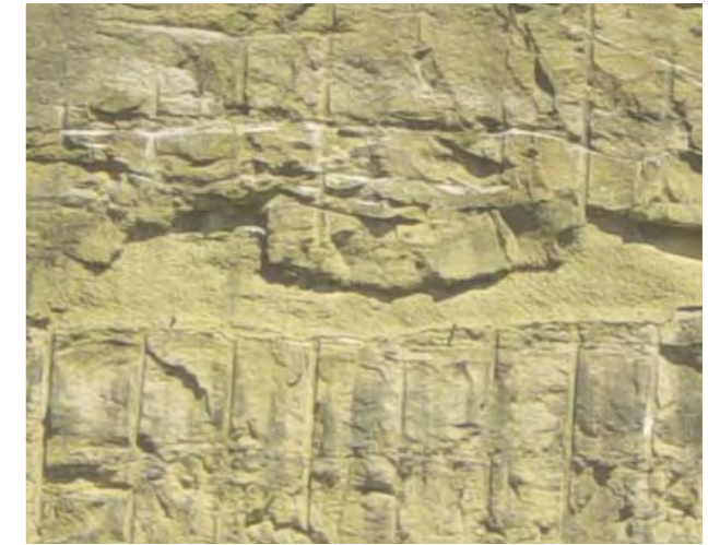
EXPOSED ROCK CUTTING WITH SEAM OF SHOTCRETE. (FROM RTA'S SHOTCRETE DESIGN GUIDELINES 2005)
